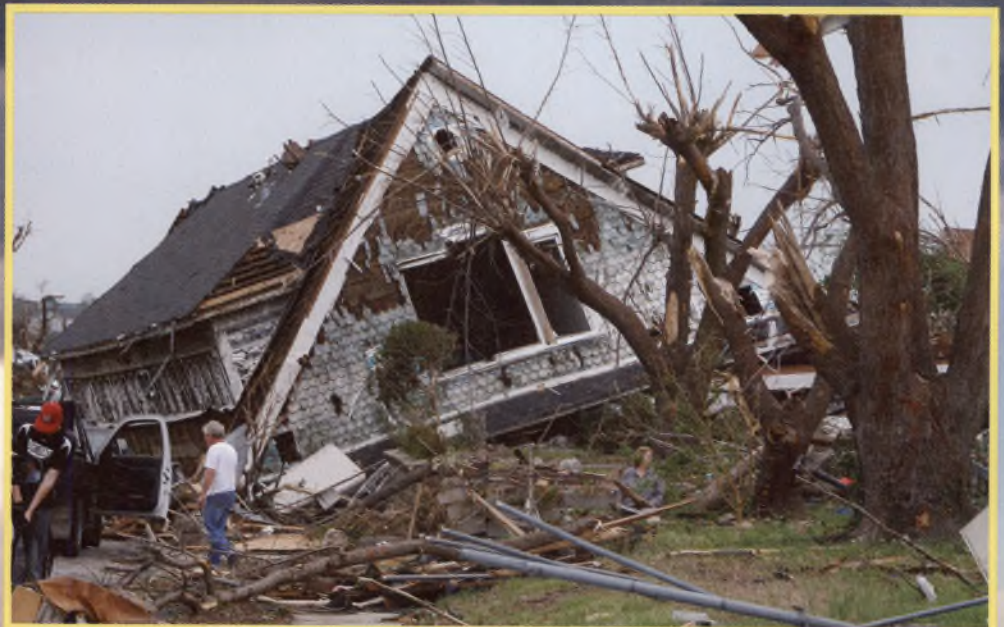
The tornado damaged this house in Joplin, Missouri.
